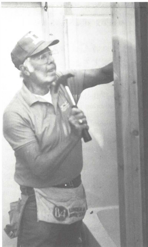
Robert Lamison (at left) and Liz and Jim Smith (below) were among Trinity members and dozens of others from the community who took part in the Thanksgiving Week Blitz Build for Habitat for Humanity. With contributions of labor and money to buy building materials, six houses will be provided at low cost to families who otherwise could not afford a home of their own.
