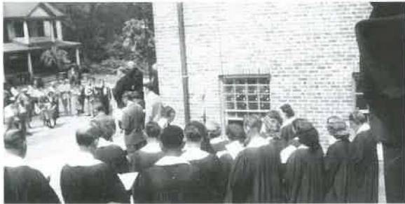
Trinity Hall Cornerstone Laying, 1949
