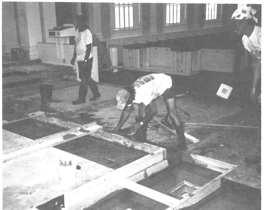
WORKMEN PREPARE CHANCEL FLOOR for Italian slate surface.
