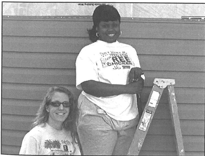
Trinity member, Deb Fadool, helps homeowner, Felicia Coleman, put up siding as construction progresses on the Habitat House.
