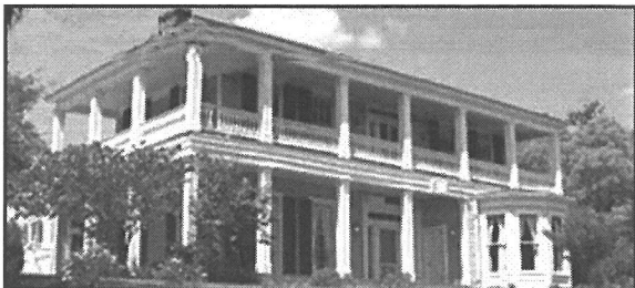
The Orman House was built in 1838 by Thomas Orman. The wood for this two story home was cut to measure near Syracuse, New York and shipped to Apalachicola by sailing vessel around the Florida Keys then assembled on the bluff overlooking the broad estuary and bay of the Apalachicola River.
