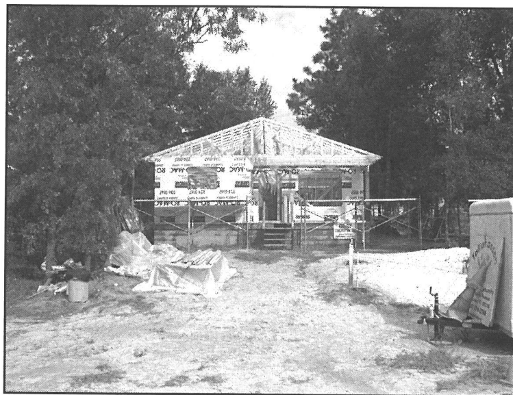
Results from Day 2 show even more progress. The roof trusses have been raised and the vapor barrier is starting to be put on the plywood exterior.
