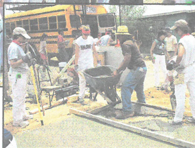
In the photo above, Vanessa Carey and Malinda Rains mix concrete for the floor slab.
