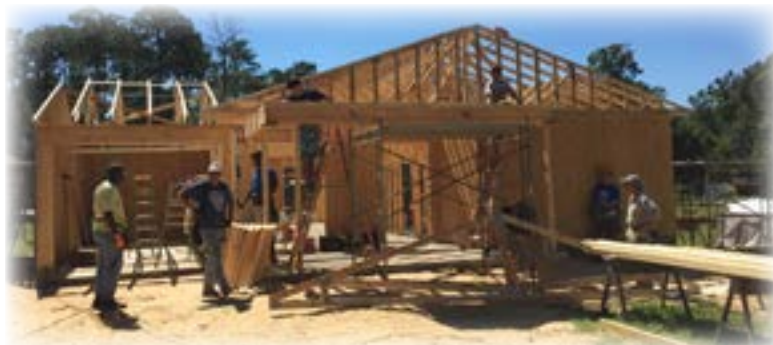
The framing is close to completion in the photo to the left. Marti Chumbler, red shirt, nails rafters to the framing.
