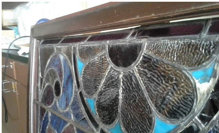
Bent bottom of window
